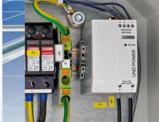
UNO DC/DC converters for direct supply of Combiner Box from photovoltaic panel
